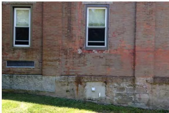
Figure S7: Poor Wall Patches
