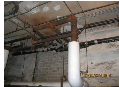
Figure P2. Heating Piping without Insulation
