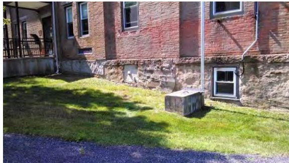
Figure C13. Poor Overland Drainage Adjacent to North Side of Building
