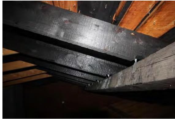
Figure S4: Charred Roof Rafters
