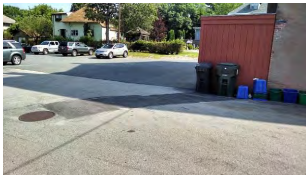
Figure C11. SMH and Pavement Patch
