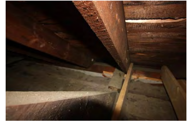
Figure S5: Damaged Truss Bearing Attic Framing Deficiencies
