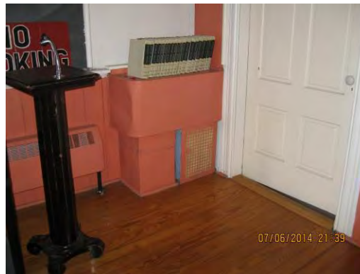
Figure P4. Ducting to Mushroom Vent
