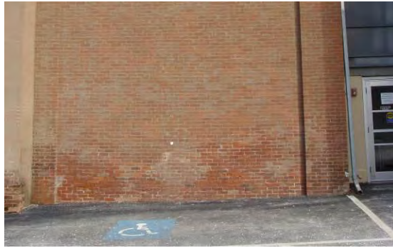
Figure S6: Deteriorated Brick Wall
