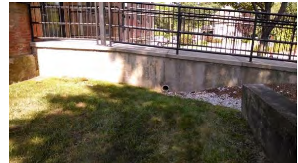
Figure C12. Poor Overland Drainage Adjacent to North Side of Building
