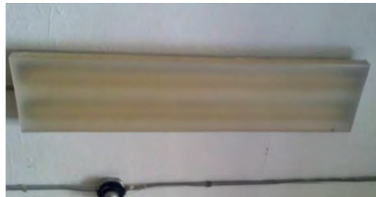
Figure P6. Lighting Fixture with Yellowed Lens
