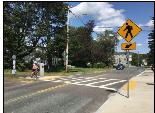
Newly constructed sidewalk on Ironstone Street
